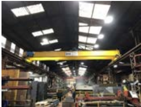
FIGURE 12 TWIGG STEELYARD INTERNAL ROOF STRUCTURE
