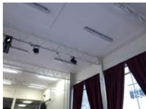
FIGURE 15 INTERNAL ROOF STRUCTURE HIGHFIELDS LOWER
