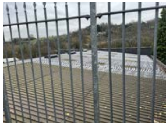
FIGURE 7-TWIGG STORES' EXTERNAL ROOF
